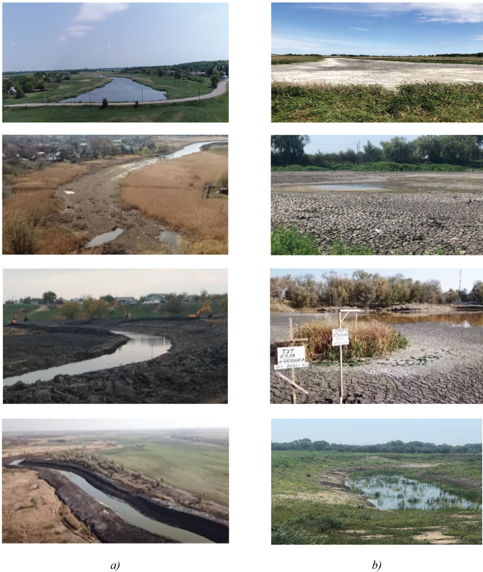
Figure 4. State of the Chaplynka River before (a) during and (b) after riverbed clearing.
