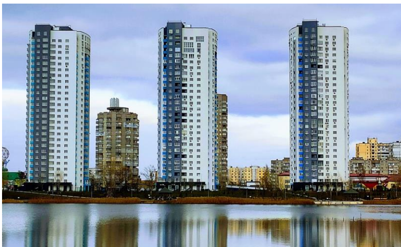
Figure 8. Photo of three 27-storey buildings built in Kiev using vibration seismic insulation.
