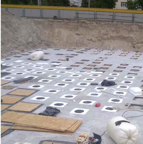
Figure 2. Installation of vibration protection system.
