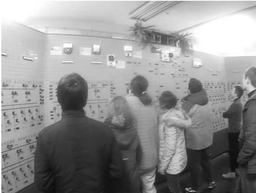
Fig.1 – A digital set of automation equipment based on the Granit telecomplex and the SinSys upgradeable software
