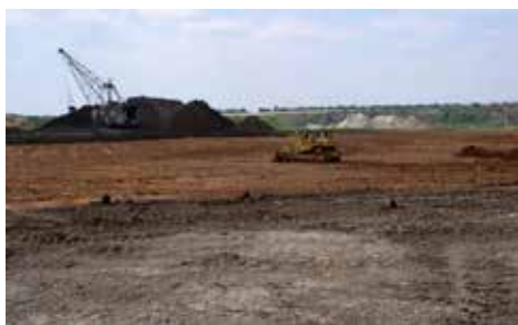
Figure 1. Leveling the surface of the field with a bulldozer
