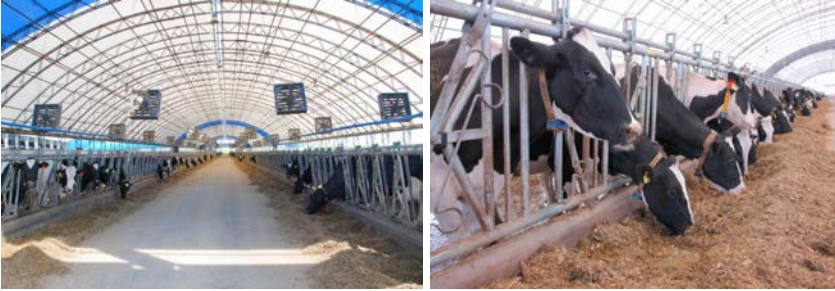
Figure 3. Non-insulated barn of hangar type with tent coating
