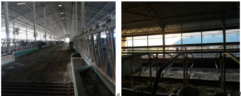
Figure 2. Lightweight premise frame for 600 milk cows: a) inside view of the premise from the side of feed table; b) boxes for cows rest
